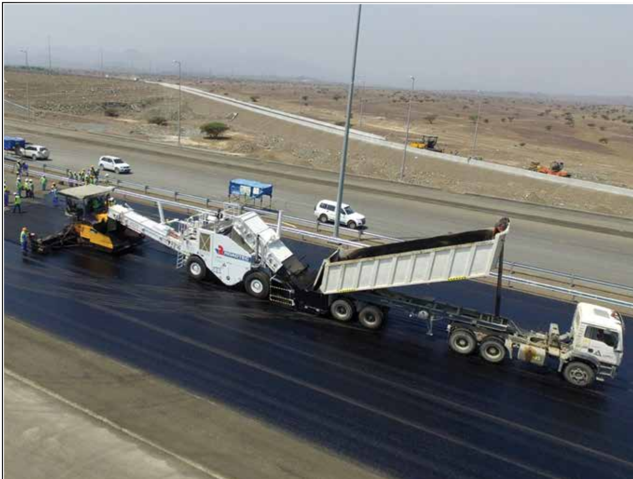
Asphalt Feeder - First Stretch
