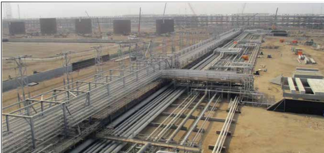
R5 Corridor: Steel Structure and pipe erection is ongoing
