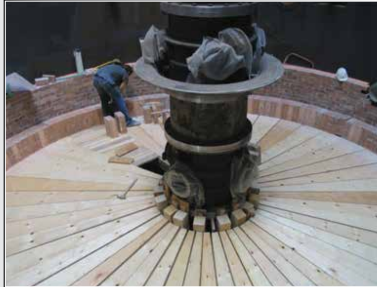
Figure 6: Hearth Refractory Installation
